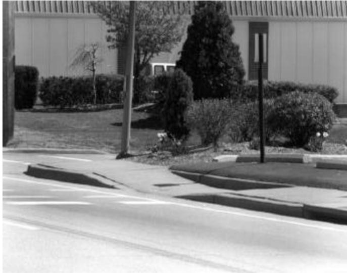
**Exhibit 4-24. Sidewalk Curb Ramp at End of Curb Radius**
