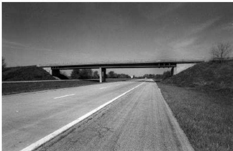
**Exhibit 10-3. Typical Grade Separation Structures With Closed Abutments**
