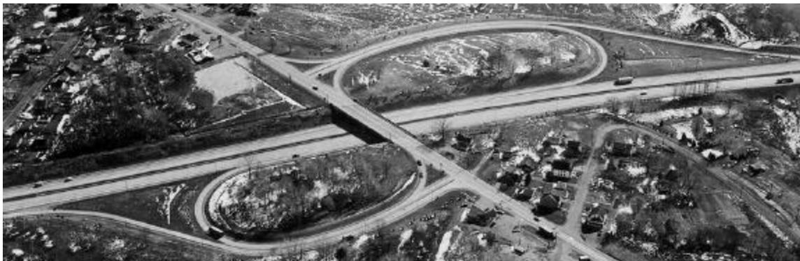
**Exhibit 10-29. Four-Leg Interchange (Partial or Two-Quadrant Cloverleaf with Ramps Before Main Structure)**
