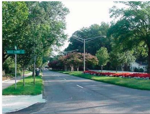
*There are a variety of median types. The medians shown above range from minimal to substantial. Functionally, they range from those that simply separate vehicular traffic movements to those that provide fully functional, aesthetic enhancements to the street. The Urban Street Design Guidelines generally discourage minimal, single-function medians.*
