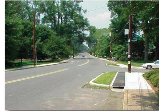
*Curb extensions can be installed as a retrofit, such as in the photo at the top, or, preferably, as part of the original design. They can also occur at intersections or mid-block, as shown below.*
