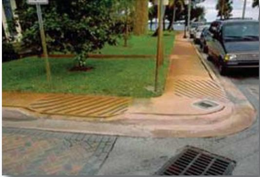
*Two radically different curb radii. The radius at the top is very small (or “tight”), which helps to slow turning vehicles. The radius below is very large (or “wide”), allowing vehicles to turn more easily and quickly. Note the location of the crosswalk relative to the curve. The radius above is more conducive to pedestrian travel. Note also the different traffic characteristics - the intersection below must handle a much larger volume of traffic.*
