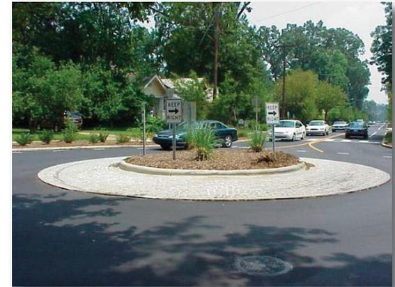
***A roundabout in a residential neighborhood, where five street segments converge. Note the “apron” that allows larger vehicles to negotiate the roundabout.***
