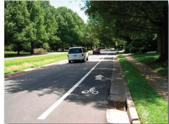
***An example of a “road diet”. This street was a four-lane street with a wide median. It was converted to a two-lane street, with bike lanes (and with the wide median remaining).***
